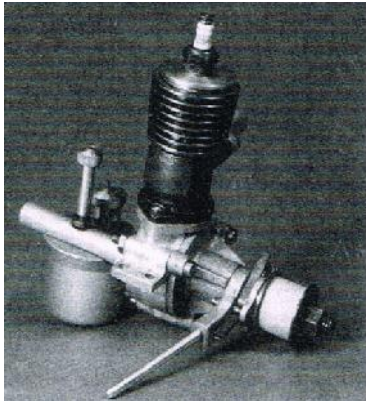
WILLARD .19 Designed and produced in small numbers in 1939 by Willard Hungerford, Los Angeles, California. First rear disc valve model engine.
