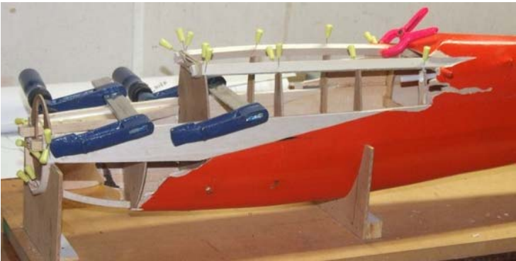
Fuselage back in building jig with crutch members spliced and five new plywood bulkheads.
