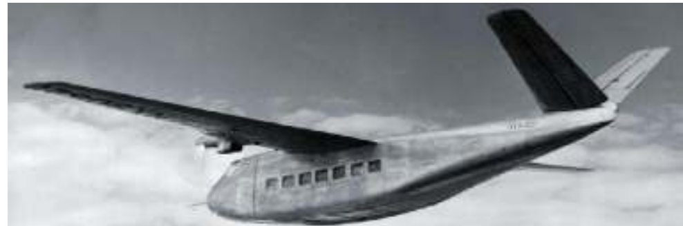
The Model 35 included a strengthened belly, which proved its worth when a fire led to a crash of the prototype on January 17, 1949. The co-pilot was killed and the pilot injured. (HistoryNet Archives)
