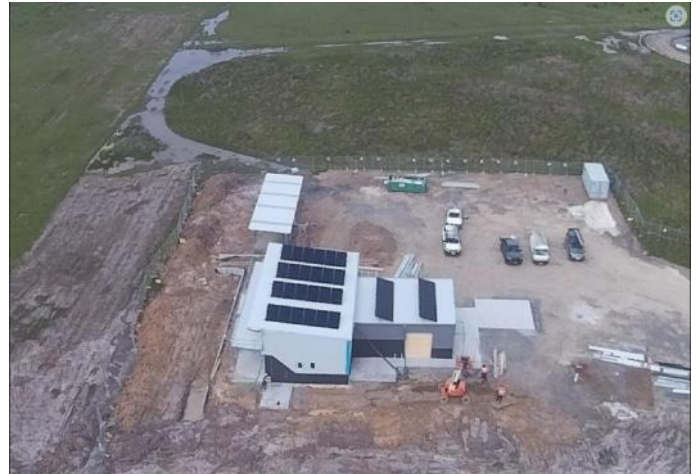
The venue will be self contained with solar panels for electric power.
