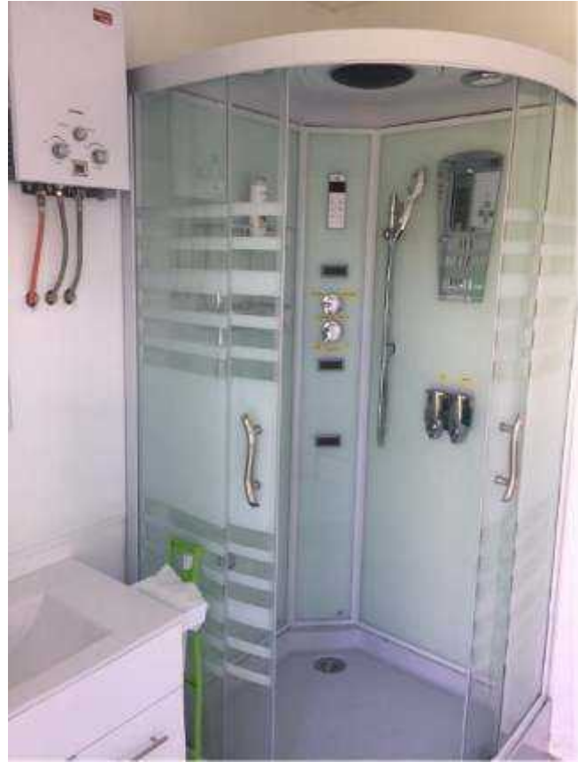
NAAS shower facility.
